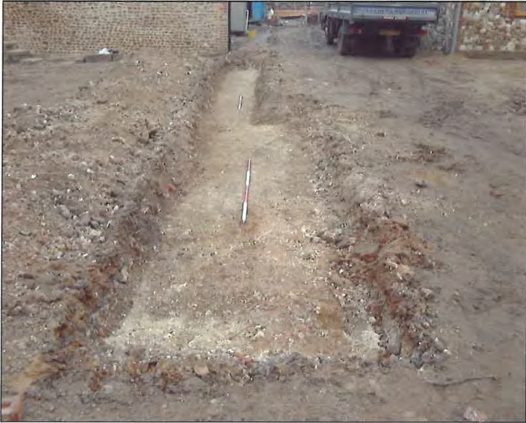
Plate 1. The evaluation trench looking north.
