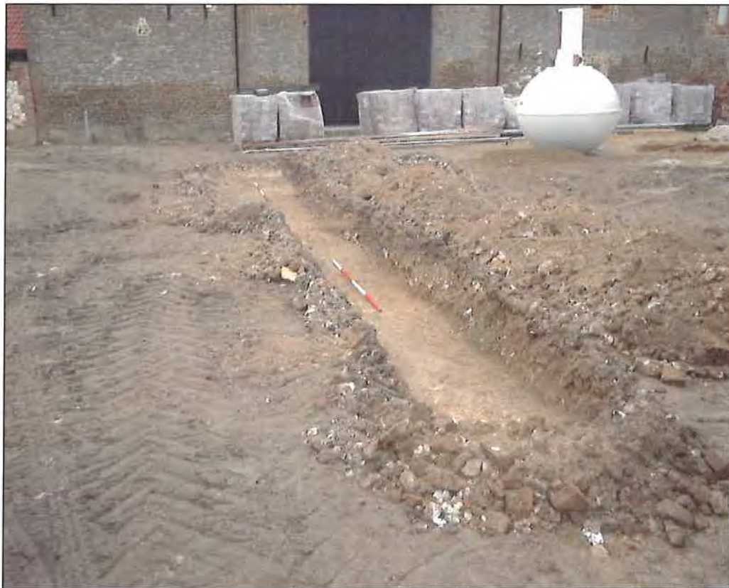
Plate 2. The evaluation trench looking south south-west.
