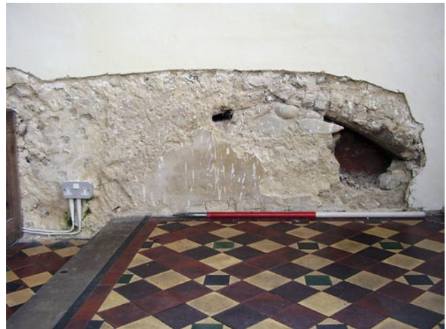
Plate 7 Wiveton, St Mary's church: exposed recess in the northern wall of the chancel.
