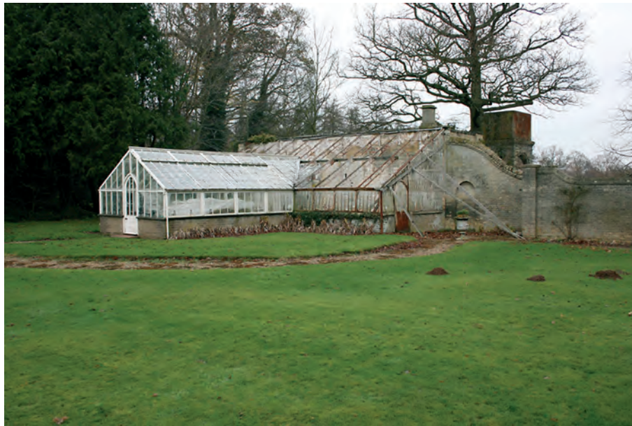
Plate 4 Hoveton Hall, Neatishead: the glasshouse from the south-east. ©NAU Archaeology.
