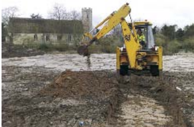
Plate 5 Filby: The site being stripped with a JCB.
